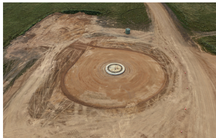
Figure 2: Backfilled turbine foundation
