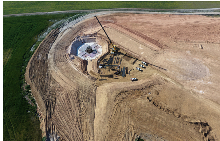
Figure 1: Workers preparing to install anchor cage in turbine
