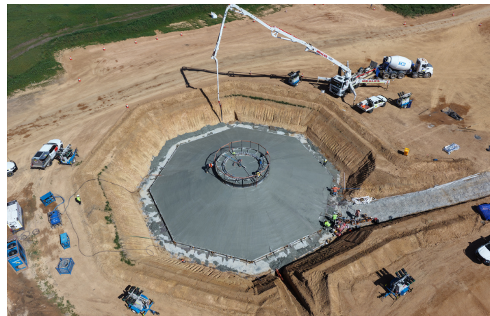
Figure 1: Aerial view of the final stages of a concrete pour
