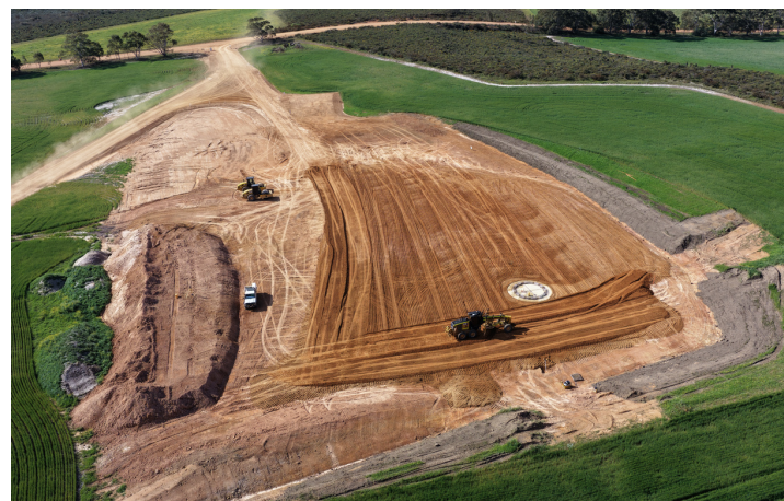
Figure 2: Workers backfilling a turbine foundation
