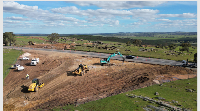
Photo: Construction of Randell Road site access points, 28 August 2026, Source: BMD
