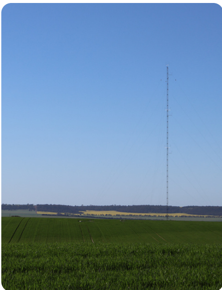
Figure 1: Meteorological mast at Waddi Wind Farm near Dandaragan
