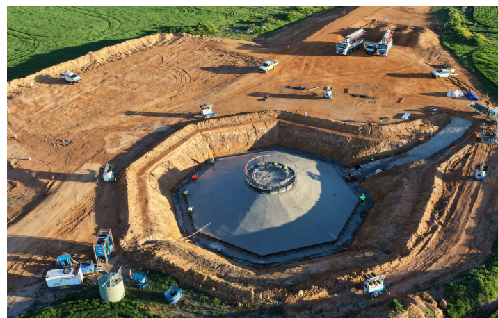
Figure 2: Aerial view of the final stages of a concrete pour
