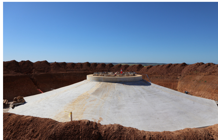
Figure 1: Concrete curing in a turbine foundation
