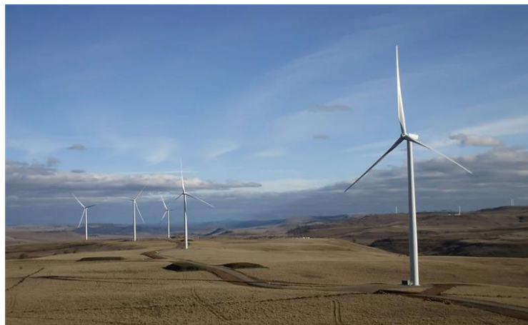
Figure 1 Boco Rock Wind Farm
