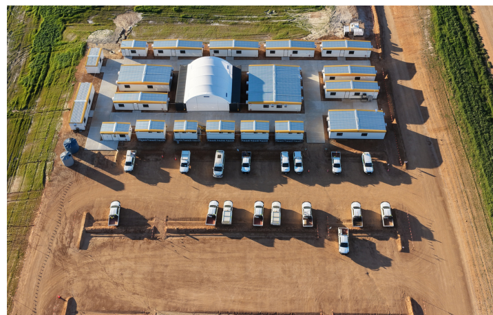
Figure 2: Aerial view of the site compound
