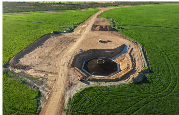
Figure 1: Aerial shot of first turbine reinforcement structure
