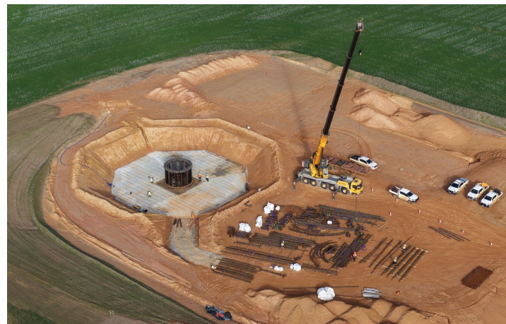
Figure 1: Start of steelworks in the first turbine foundation
