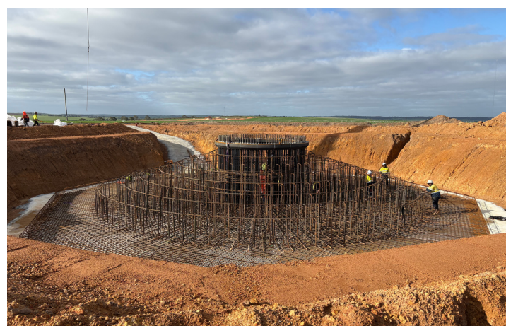
Figure 2: Anchor cage taking shape in the first turbine foundation
