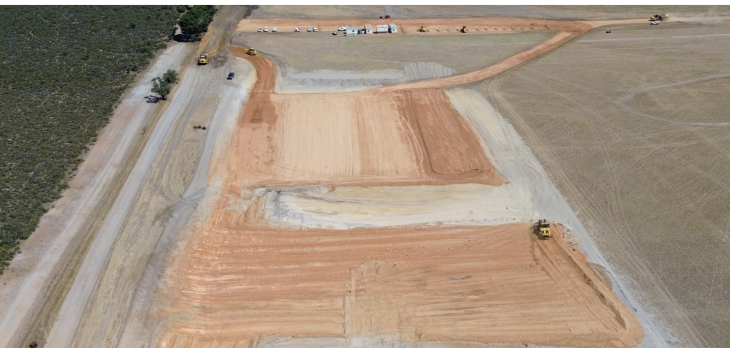
Figure 1: Preparing the site compound and concrete batching plant area at Waddi Wind Farm
