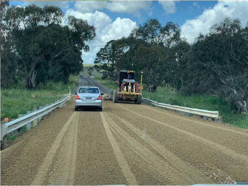
Hardiman Creek during emergency repairs
