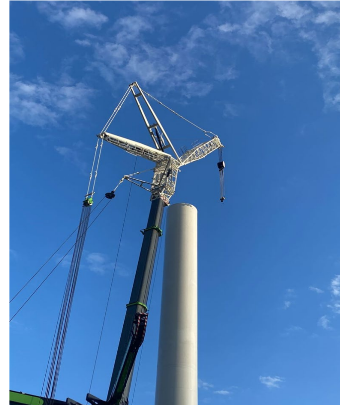
First Base and 2 tower sections installed
