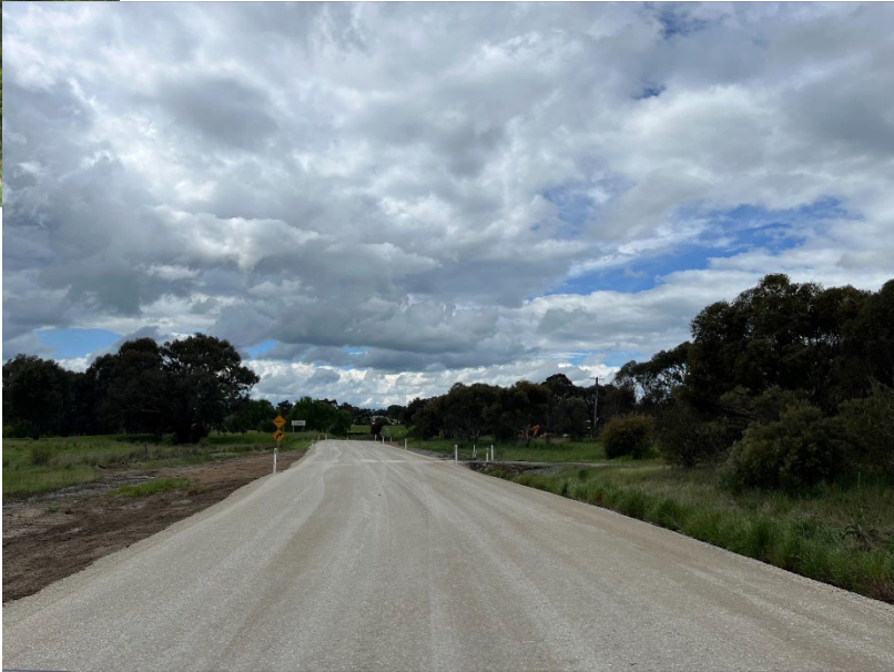
Trucking Yard Road after emergency repairs
