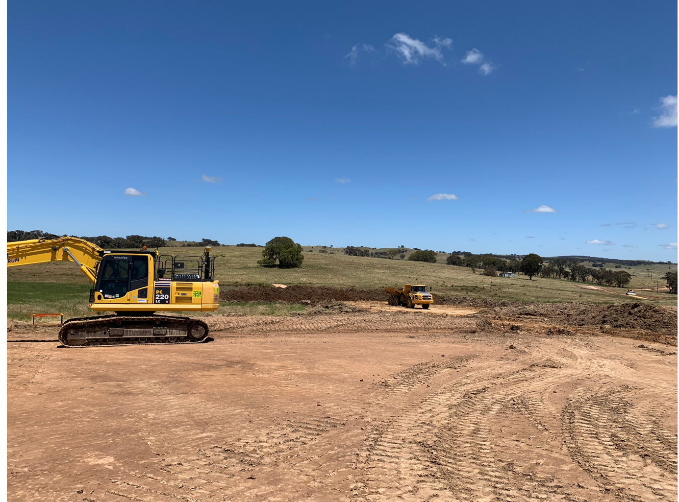
Earthworks commenced on temporary site compound
