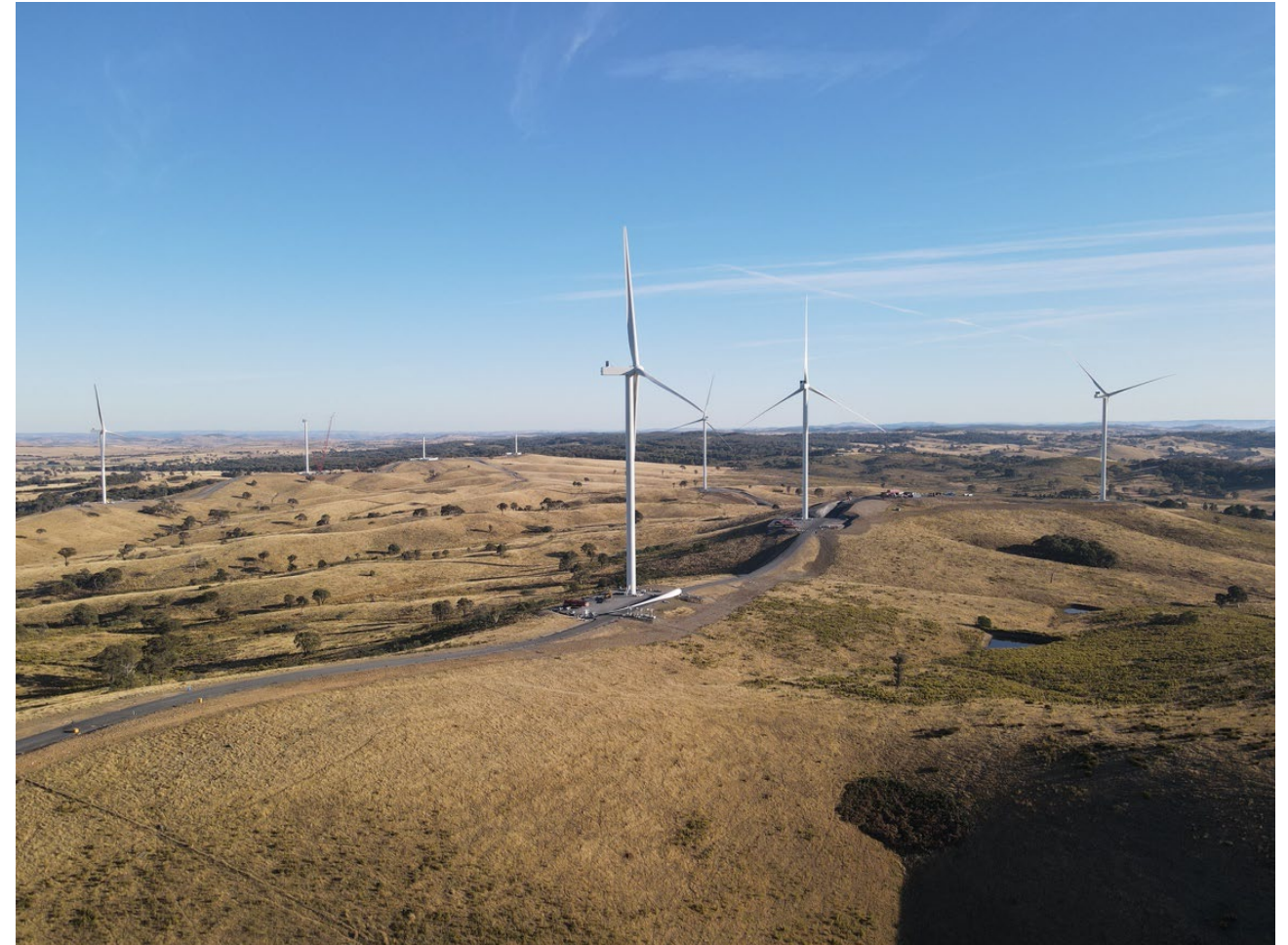
WTG A07 looking north
