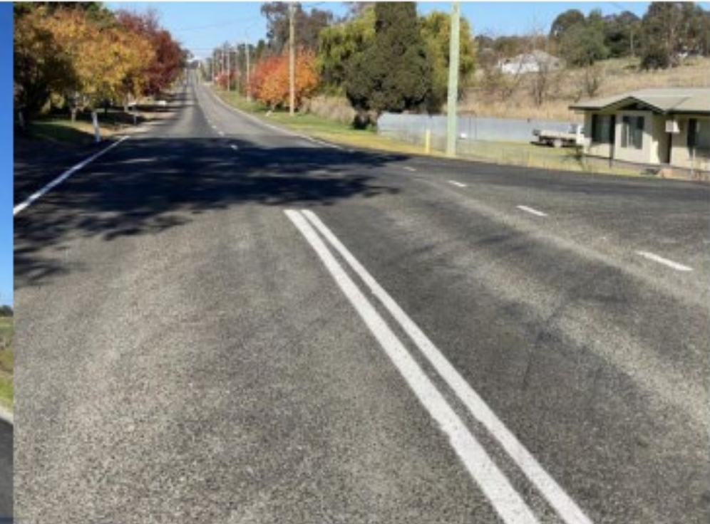
Completed Yass Street / Boorowa Road intersection
