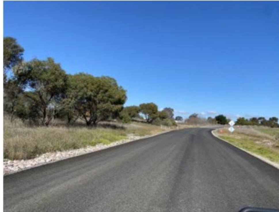
Resealed Trucking Yard Road
