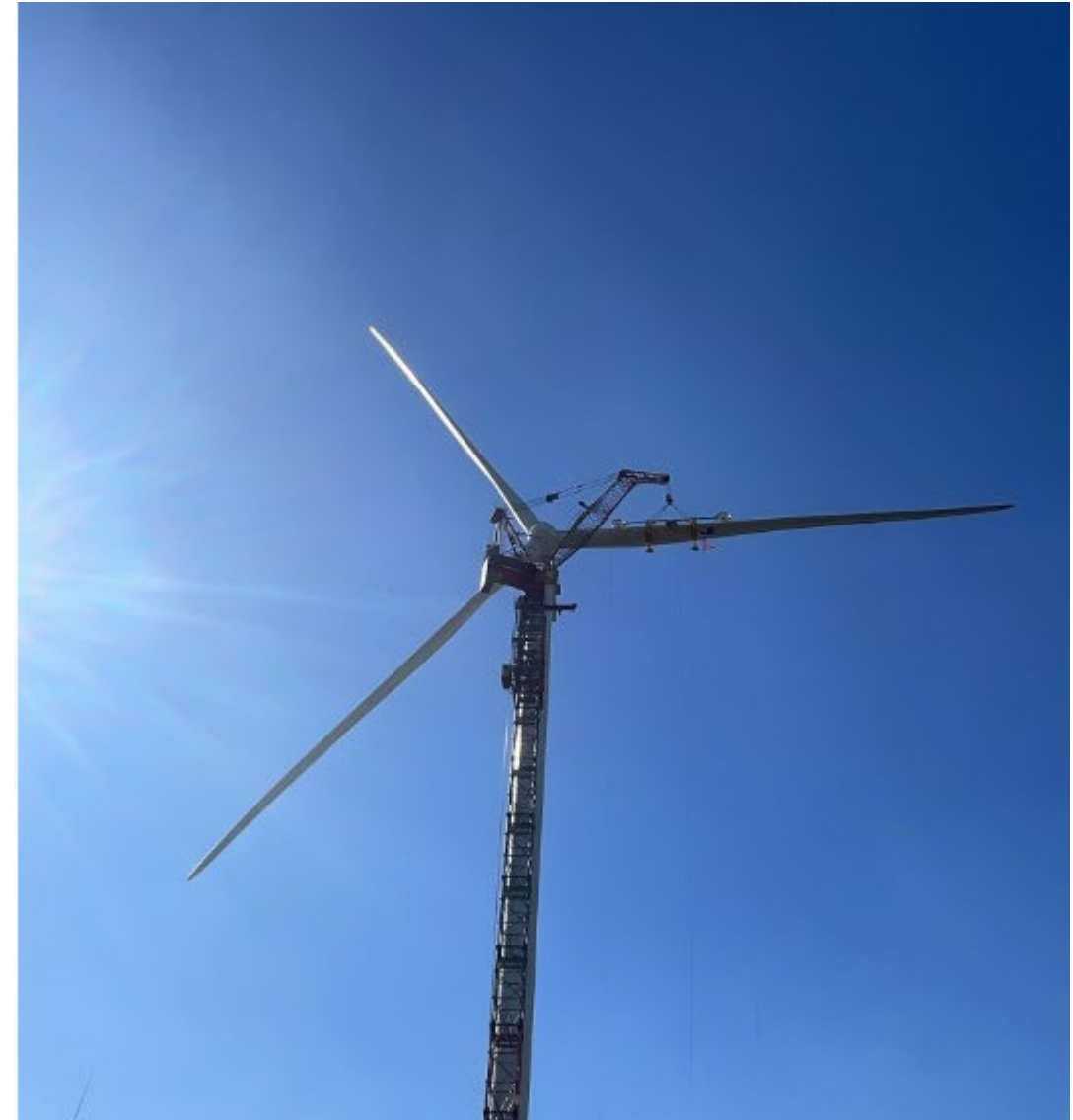
Last turbine blade installed 16 April 2024
