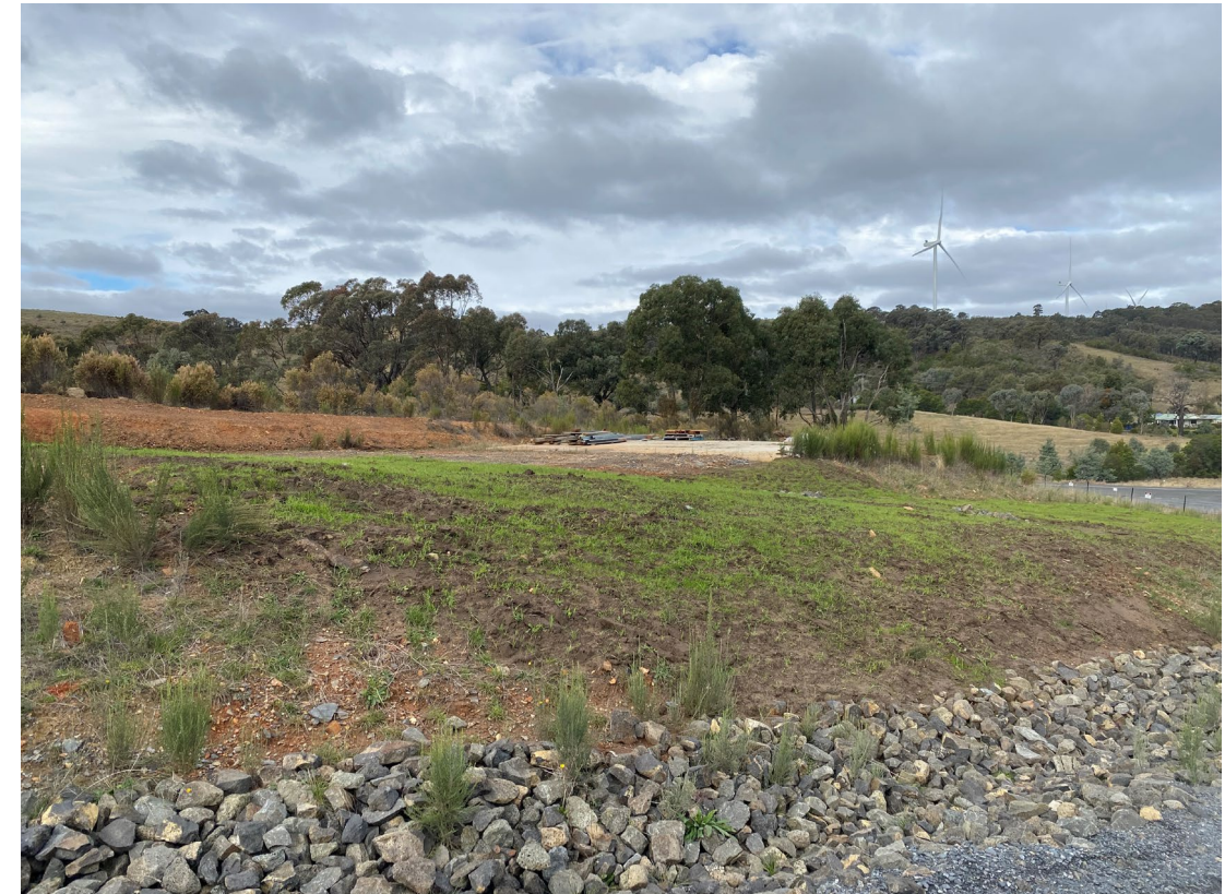
Wind farm rehabilitation taking shape
