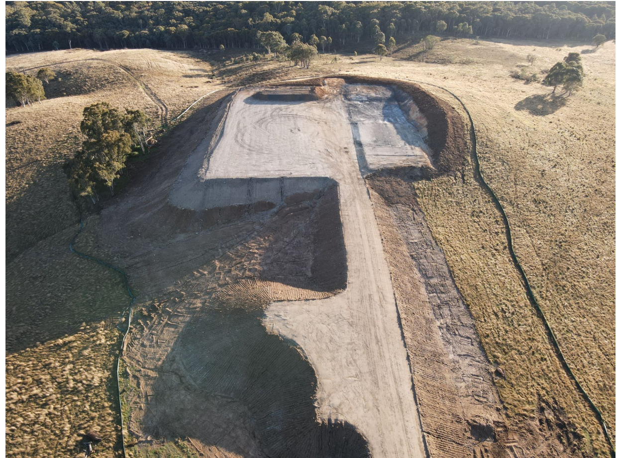
WTG hardstand construction
