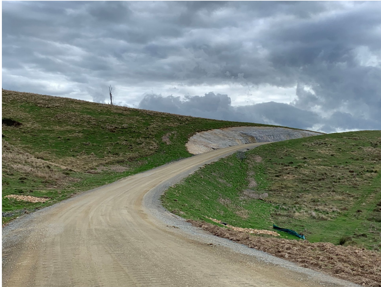
Completed wind farm access track and rehab
