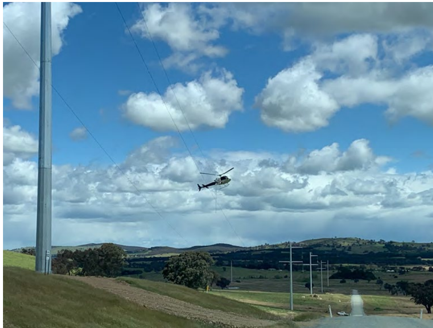
330kV Overhead Line using a helicopter
