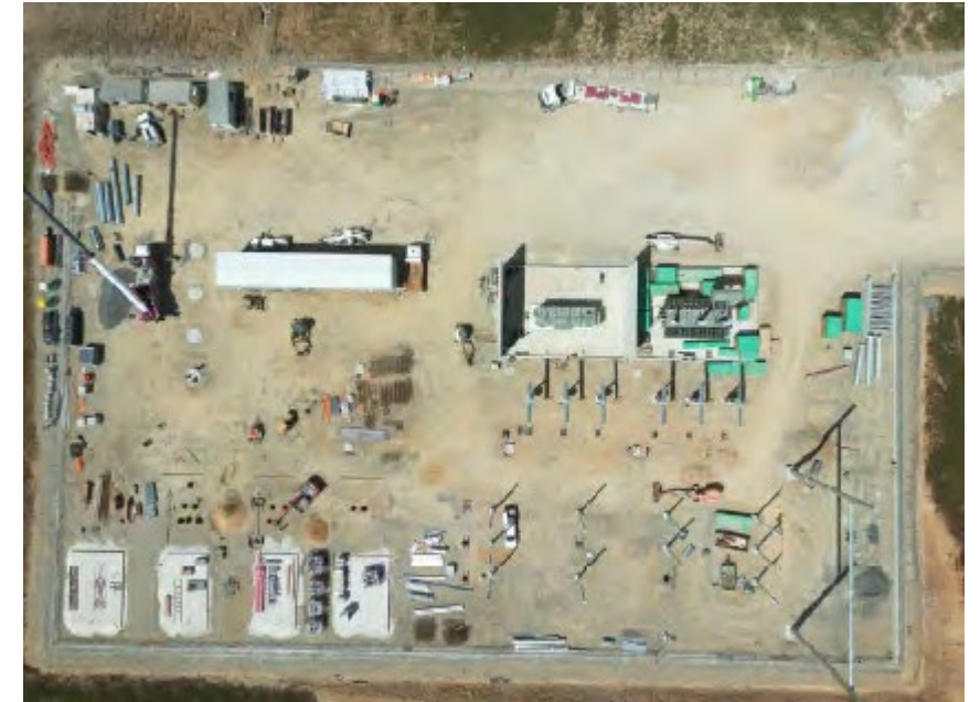
Northern Substation Progress
