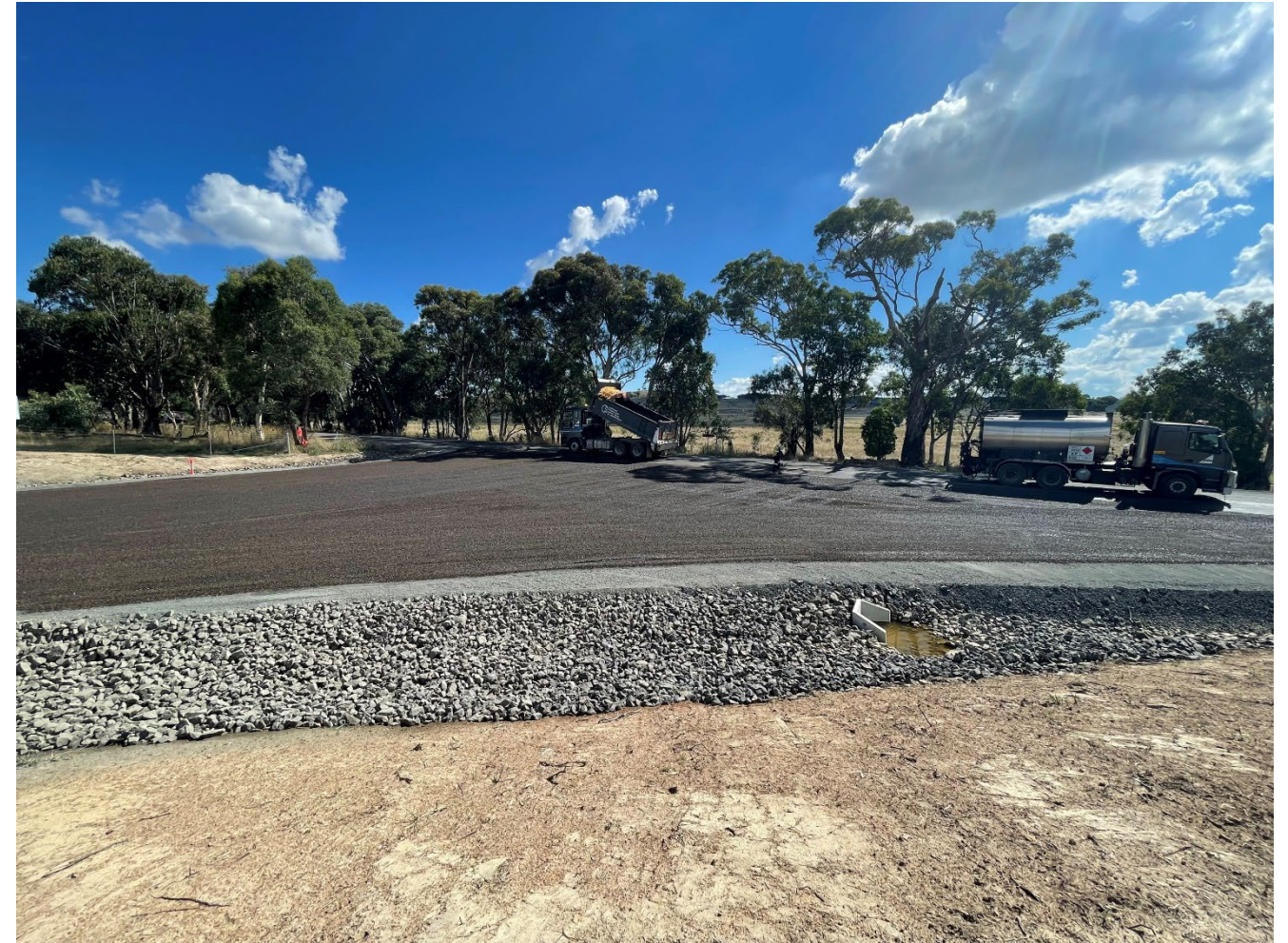
Wind Farm main entry being sealed
