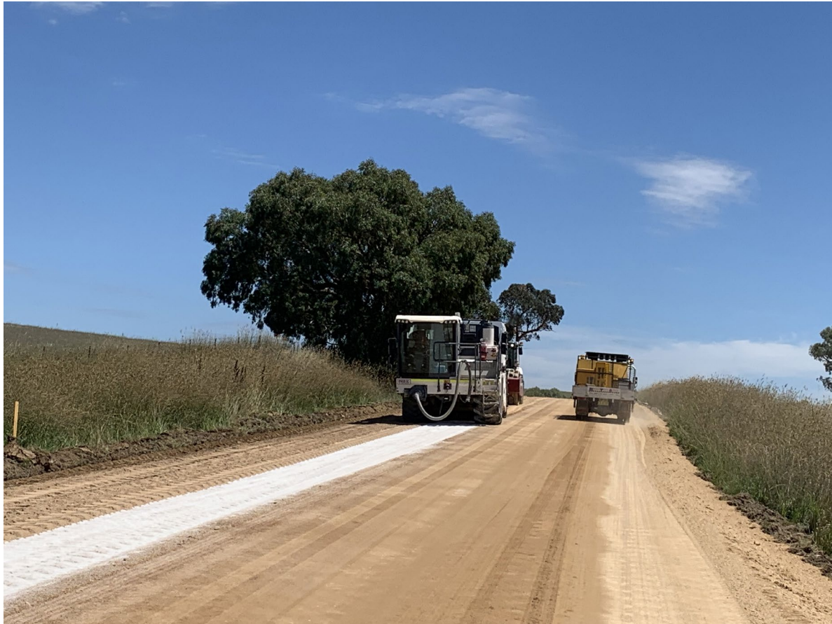
Lime stabilisation of Boorowa-Rye Park road
