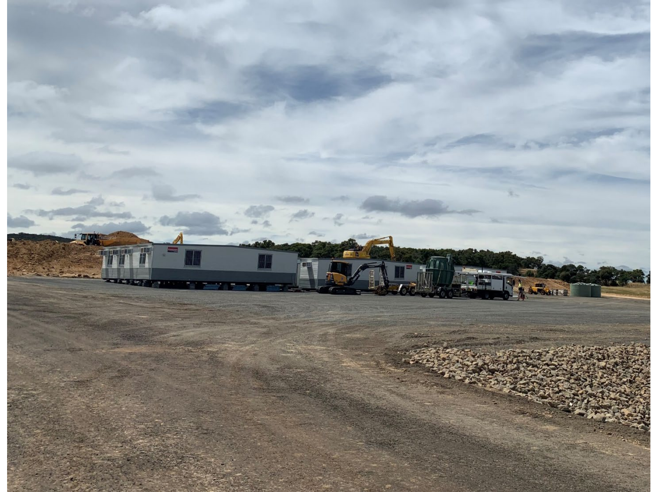
Site office being dropped at temporary compound
