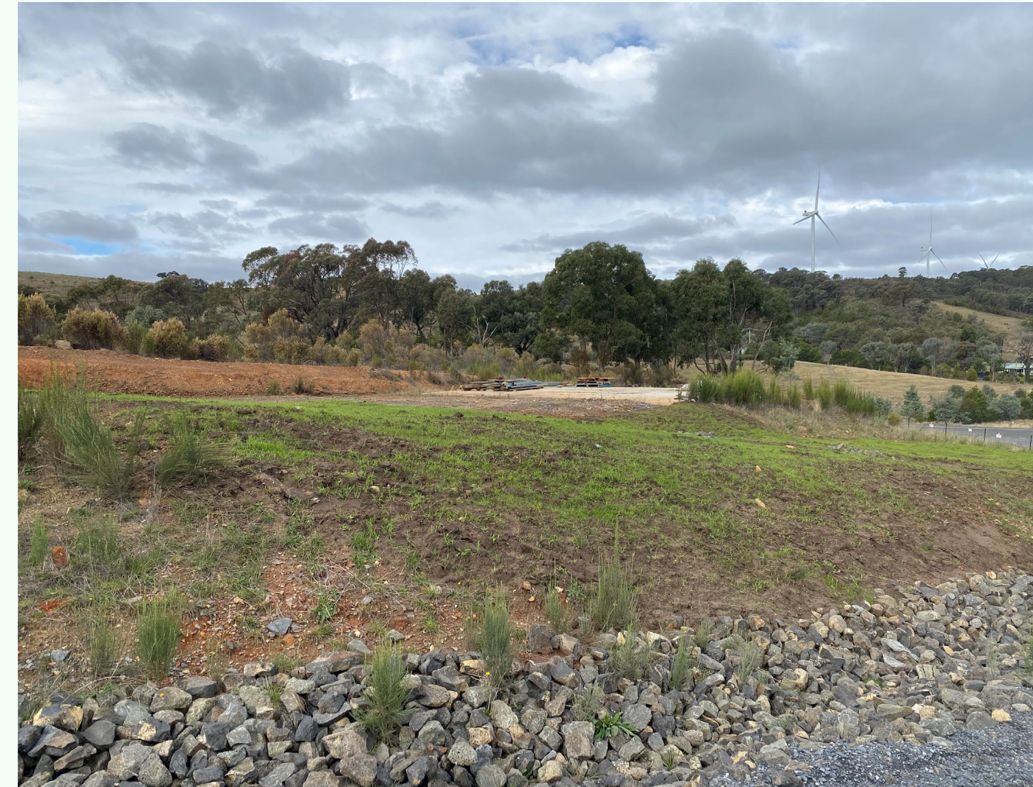
Wind farm rehabilitation taking shape.
