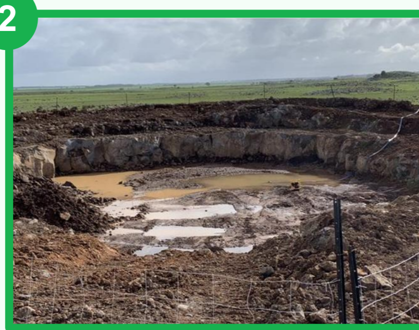
2 Civil works (access tracks, hardstands and turbine foundations)
