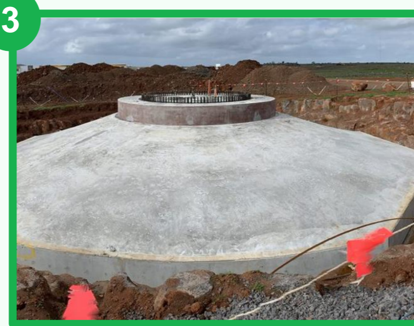
3 Pouring turbine foundations
