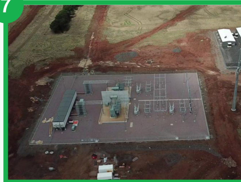
7 Electrical works (stringing the transmission line, substation works)
