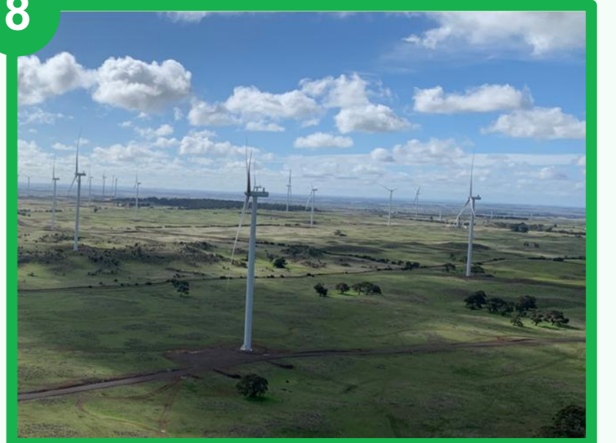
8 Testing, commissioning and finishing works
