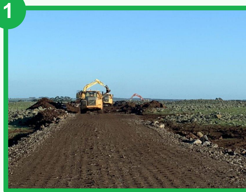
1 Early civil works (substation works and transmission access tracks)
