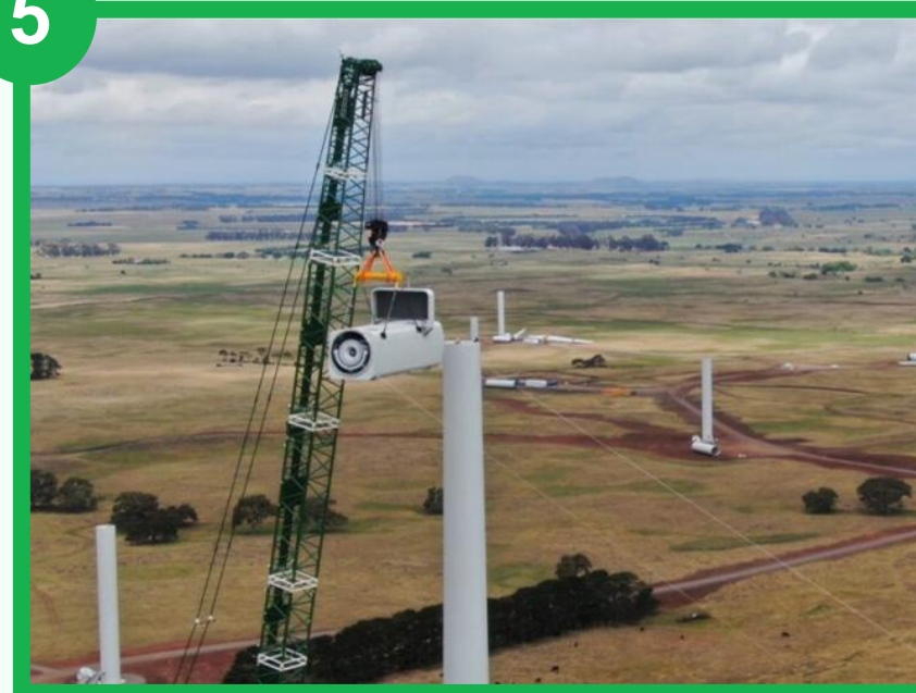
5 Setting the nacelle (or the 'brains' of the turbine)
