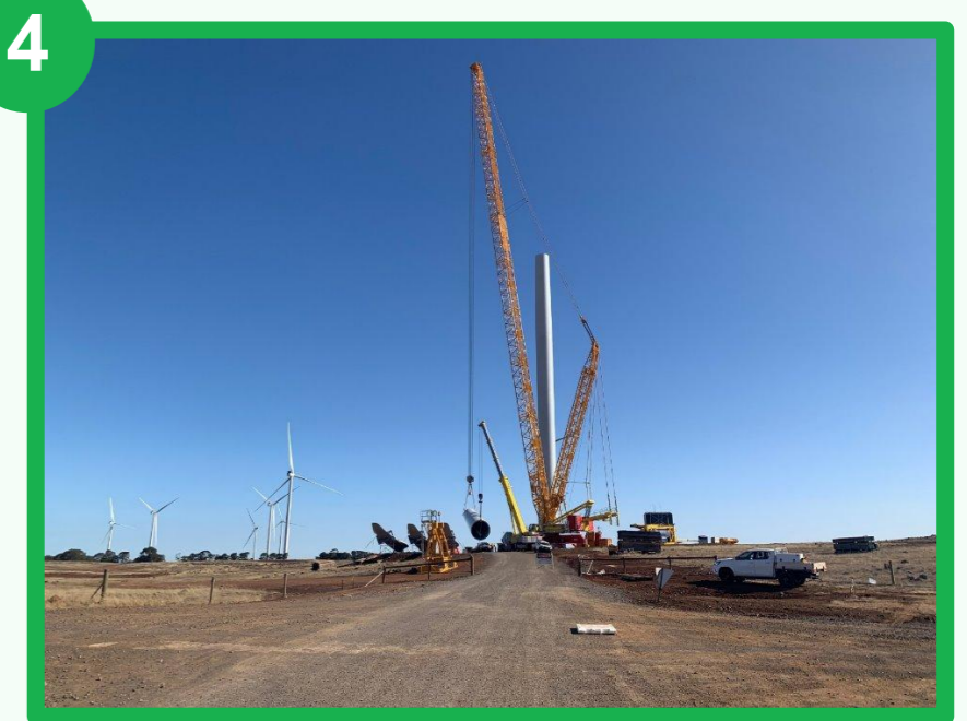
4 Turbine tower construction
