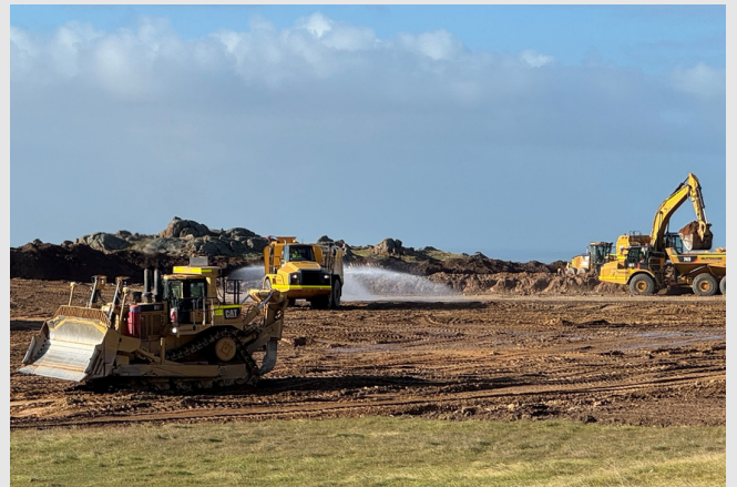
Photo: Preparing the sub-base of the site compound
