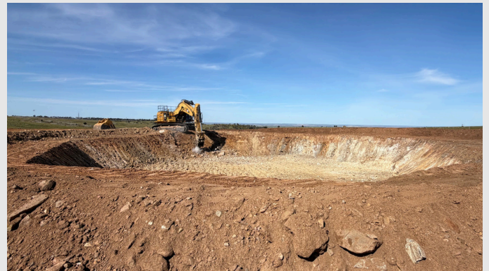
Excavation of the first turbine foundation, source: BMD
