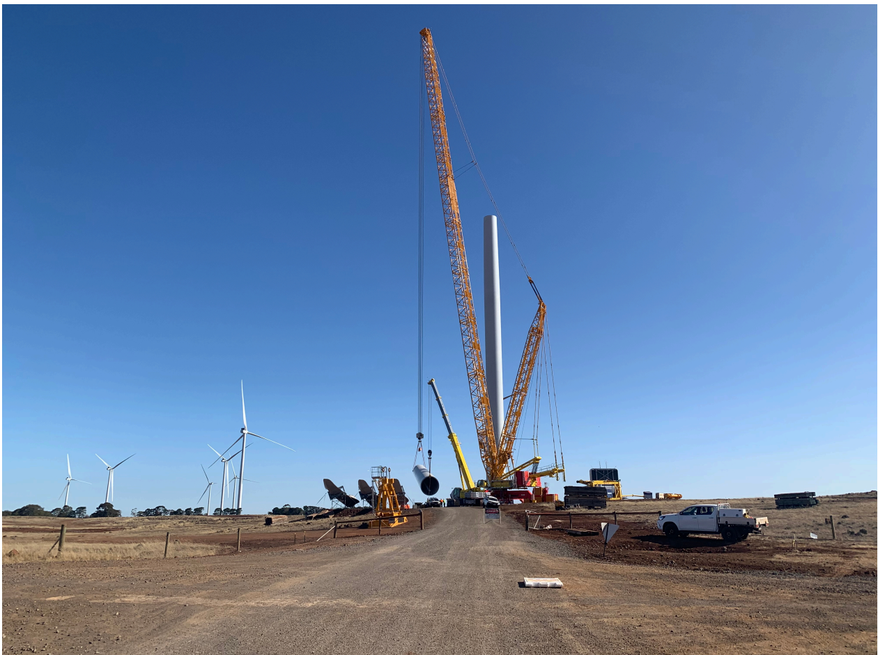
Figure 3: A crane erecting a turbine at Dundonnell Wind Farm.
