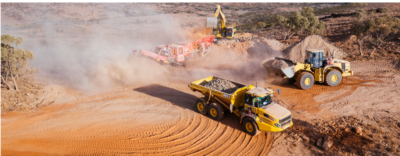
Figure 1: An example of dust created when constructing a hardstand.
