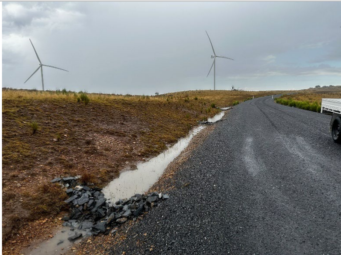
Photo 9: Rock check sediment controls and sealed access road
