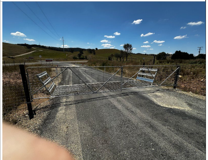
Photo 12: Stabilised site access and rumble grid
