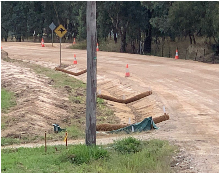
Photo 3: Erosion and sediment control, progressive installation
