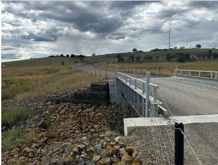
Photo 15: Upgraded bridge and waterway scour protection
