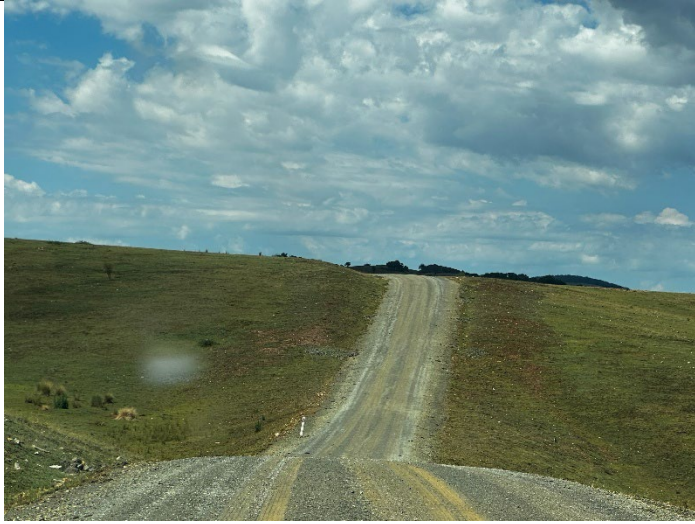
Photo 13: Graded internal access road and rehabilitation
