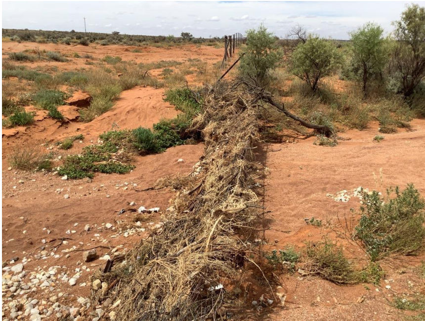
Plate 15: Fence pushed over by water and debris on the northern boundary.
