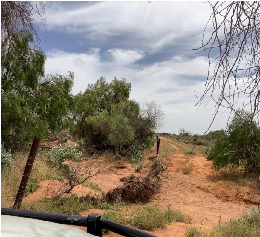
Plate 16: Fence pushed over by water and debris on the eastern boundary.
