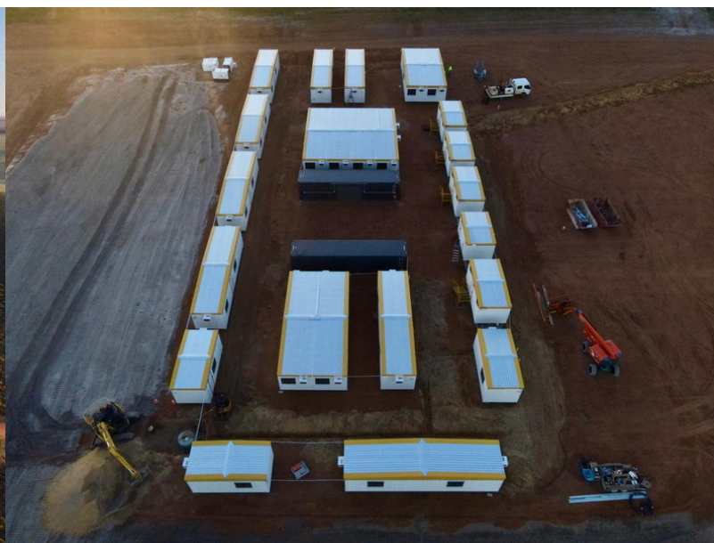
Figure 2: Aerial view of completed site compound bench and site offices
